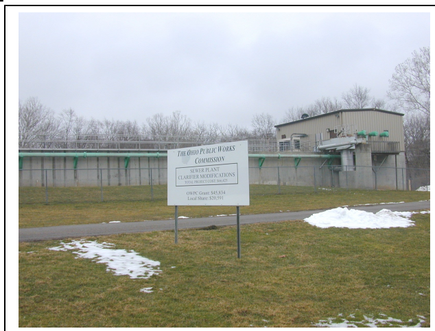
New Richmond Wastewater Treatment Plant
