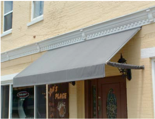
This awning has a traditional pipe frame and open ends. It is appropriately scaled to its storefront.
