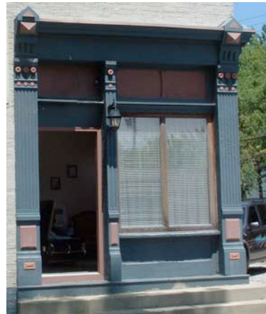
This cast iron storefront has all its basic elements intact: bulkhead, display window, transom and cornice.
