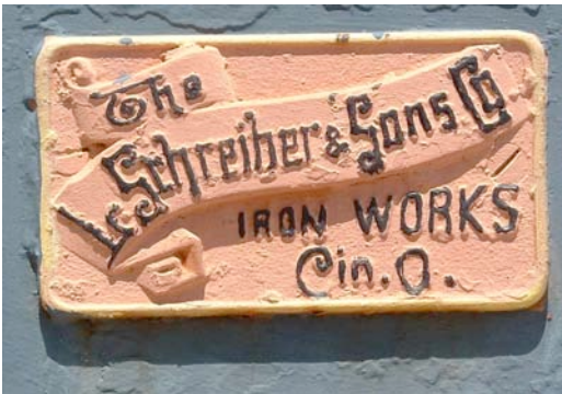
New Richmond is fortunate to have an original cast iron storefront with its builder's plate.
